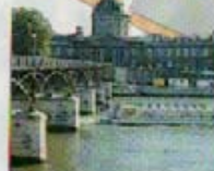
The Passerelle des Arts is a steel reconstruction of Paris's first cast-iron bridge (1804), and was inaugurated in 1984.
